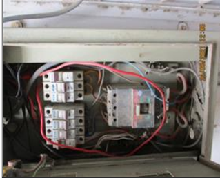
External photo(s) of the production unit(s) Loose wiring near hydrant.JPG
