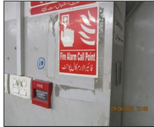
External photo(s) of the production unit(s) Fire alarm call points provided.JPG
