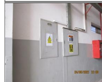
External photo(s) of the production unit(s) Hazard signs provided on electric panel.JPG
