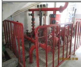
External photo(s) of the production unit(s) Fire hydrant system.JPG
